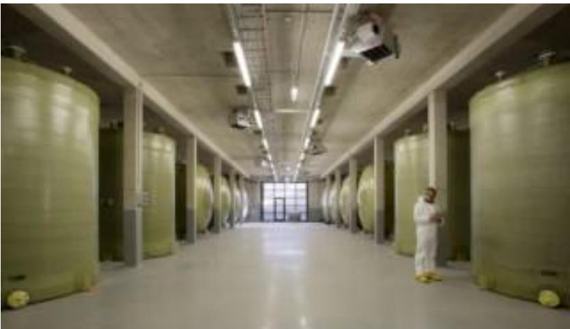
20 MWh all vanadium redox flow cell for stationary applications
